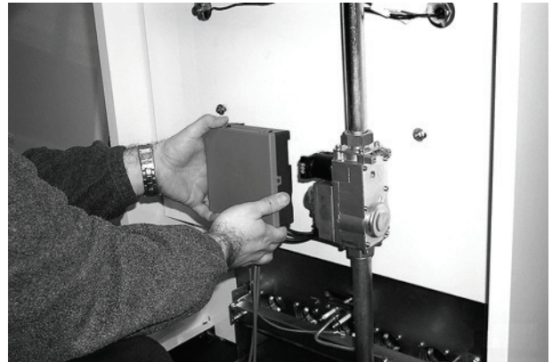
fig. 8 - Remove the control unit
